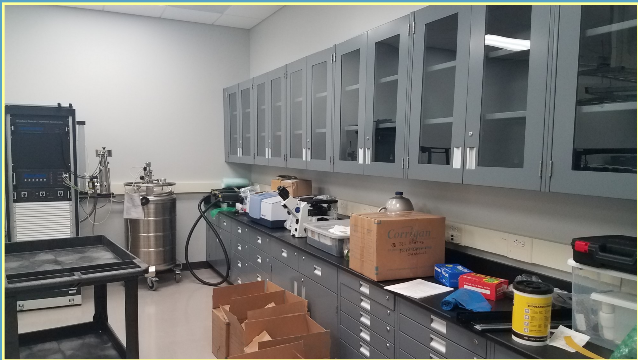
Prof. John Keiffer's Lab Renovation in Dow
